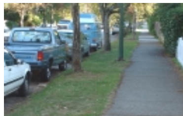
No curbs and vegetation buffer strips along Blenheim St.: runoff is slowed down and absorbed.
