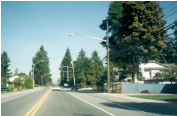
Figure 2: Cable Configuration. As shown in the photograph taken within the study area (Figure 2), many of the electricity cables are above ground. There are also underground cables present in some parts of the study area.
