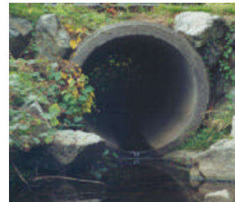
Bridges can be an appropriate design alternative in certain areas. Note the low water flow in culvert. It's doubtful fish can survive in this.
