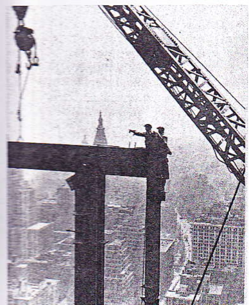
Fig. 27.24 New York, the Empire State Building under construction; a photograph by Lewis Hine entitled "Laying a Beam, Empire State Building, 1931."
